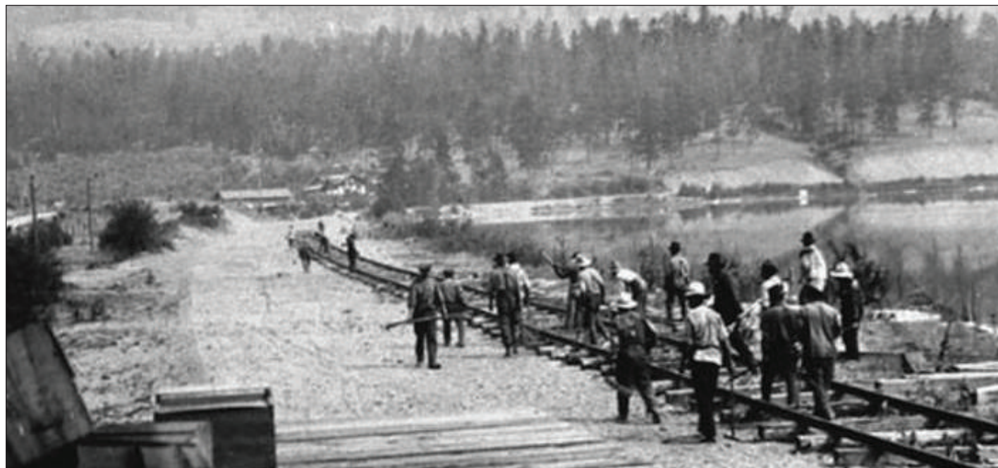
A group of workers construct the railbed of the Kelowna Line of the CNR beside Kalamalka Lake circa 1922. (Oldphotos.ca photo)
